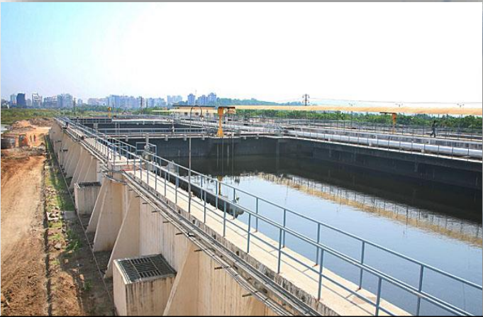
Sewage Treatment Plant, Nerul, Navi Mumbai
