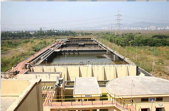
Sewage Treatment Plant, Vashi, Navi Mumbai
