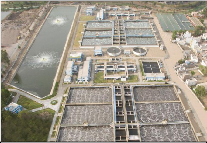
Sewage Treatment Plant, Indore
