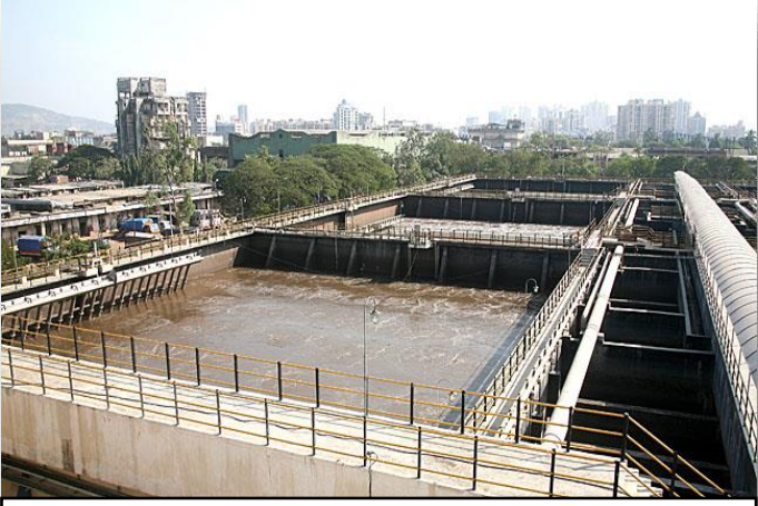
Sewage Treatment Plant, Airoli, Navi Mumbai
